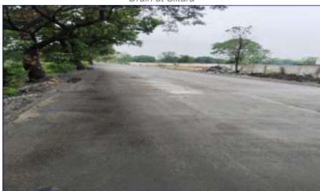
Concrete Road at Raigarh
