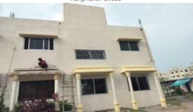
Arbindo School Construction, Kachana
