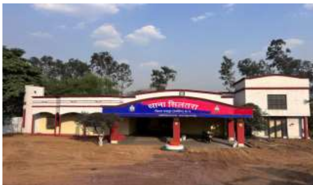
Siltara Thana Painting work
