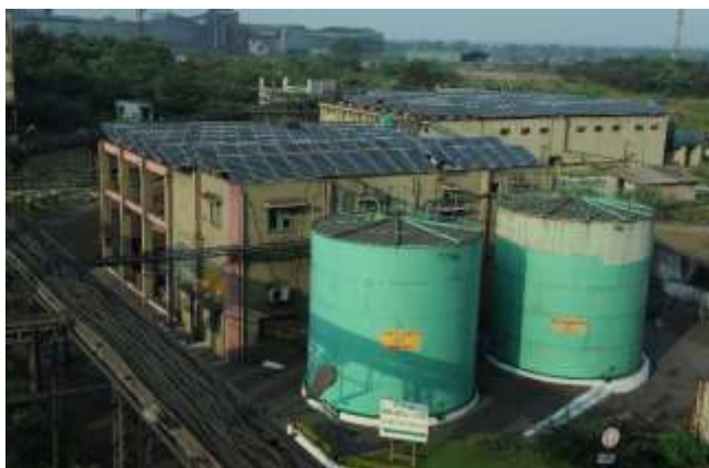
SEML Ferroalloy Production Facility, Siltara, Raipur
